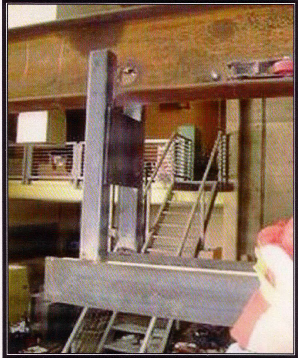
Figure 3.6- Out of Plane Bracing Photo
