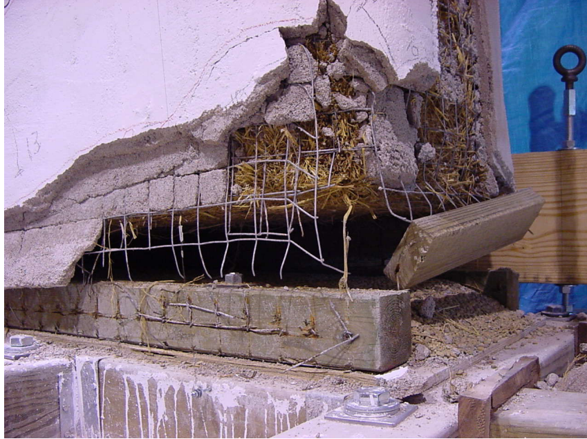
Figure 6.9 – Wall E mesh failure (7.5% drift level)
