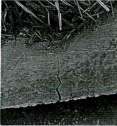
4.3F BENDING CRACK IN TENSION FACE PLASTER
