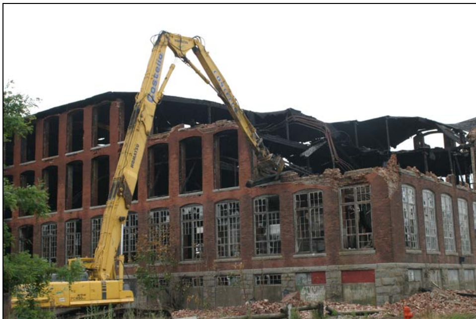
Photo courtesy of Costello Dismantling
